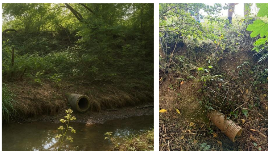
Figure 8: Outfalls for the two main collector drains shown in Figure 7b. Note the outfall shown the left image is coming out of the bank of the stream visible in the right image.
