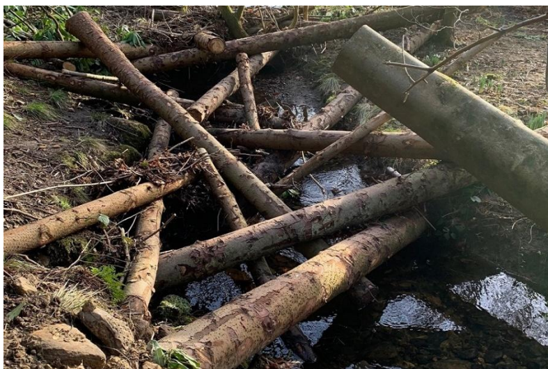
Figure 14: An example of a 'kerplunk' woody debris installation 12 .
